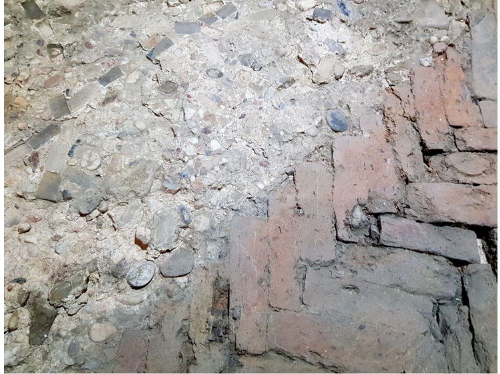
Figure 4.1 There are triangular gaps where the opus spicatum meets the mortar floor (source: K. Peterse).
