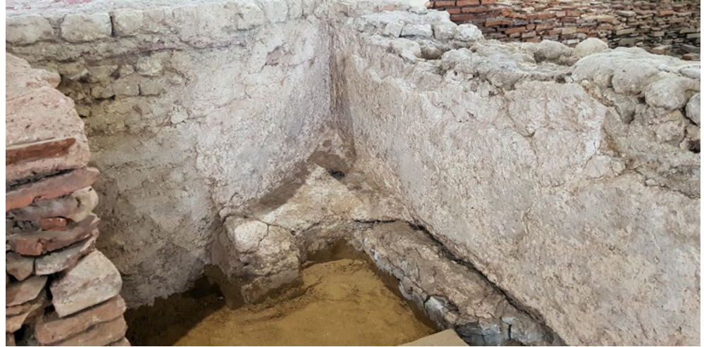
Figure 4.8 Secondary plasterwork on the west wall of the tepidarium and on part of the circular wall of the laconicum . The plasterwork was applied to prevent rising damp (source: K. Peterse).
