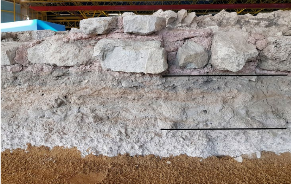
Figure 4.18 East side of the natatio . From the bottom: to the lowest black line: secondary bottom of the natatio ; between the two black stripes: backfill on secondary bottom; above the top black line: west wall of drain (source: K. Peterse).
