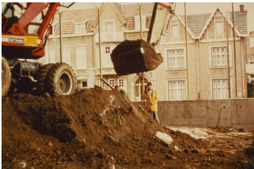
Figure 1.16 The exposure of the Roman baths in 1977. The digger was positioned above the apodyterium (source: Thermenmuseum archives).
