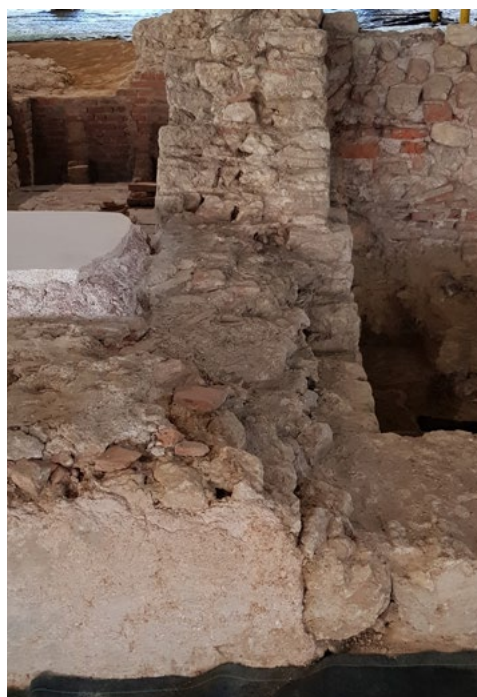
Figure 4.13 The damp-proof plasterwork on the west wall of the heated rooms ended at the transition from the alveus to praefurnium I (source: K. Peterse).
