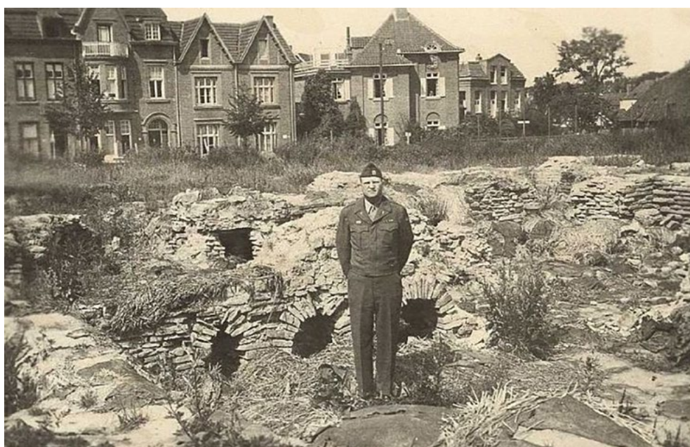
Figure 1.13 The Roman baths shortly after the liberation, with an allied soldier standing in the caldarium . The straw and tar paper can be seen in a number of places (source: Thermenmuseum archives).
