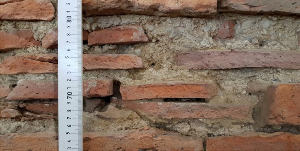
Figure 4.7 The mortar in the masonry of the tepidarium has varying (source: K. Peterse).
